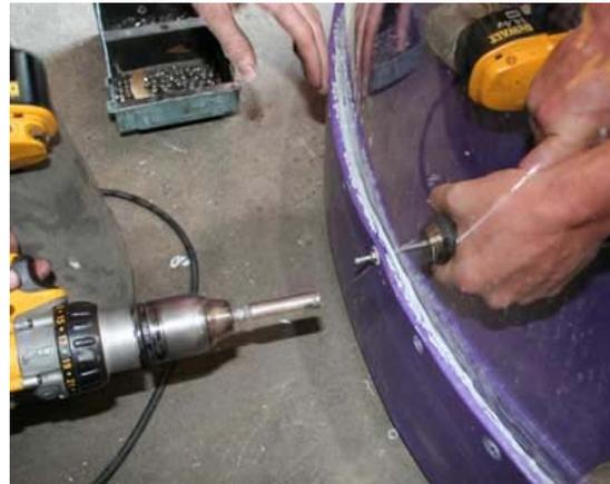
***NOTE:*** Be sure to tighten the nylon nuts snugly, but not so tight that the bolt breaks. Space each bolt approximately 3" apart, all the way around the window. After the bolts are installed, go back around and re-tighten each bolt so they are all snug and tight.
