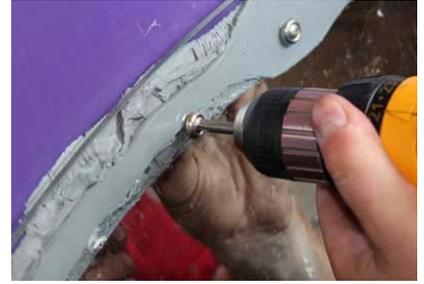
From the inside, insert the bolt with neoprene washer and finishing washer (provided) through the hole and hold it in place with a Phillips head screw driver. From the outside of the tank, place the flat washer next to the tank, and then tighten the nylon locking nut (provided).
